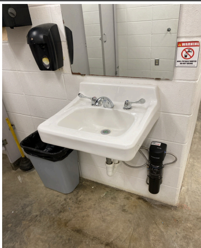
12/9/2024 - 200-27 - Malta Bend - Girls Gym Restroom
