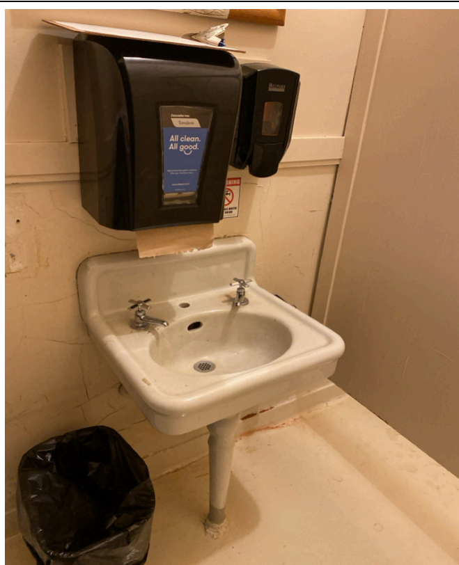
12/9/2024 - 200-21 - Malta Bend - Women's Restroom
