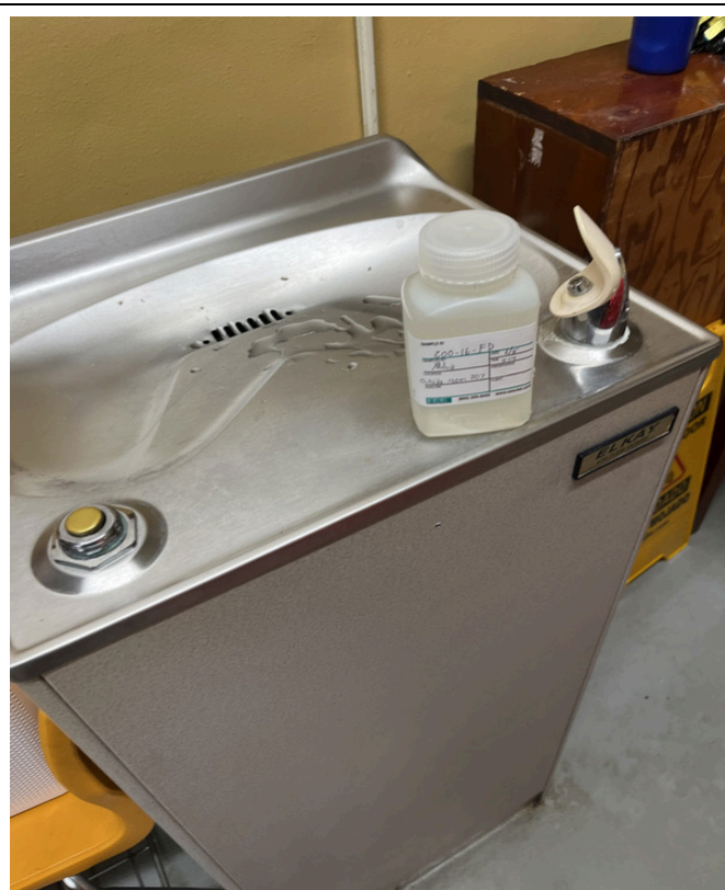
6/5/2024 - 200-16 - Malta Bend - Outside Room 207
