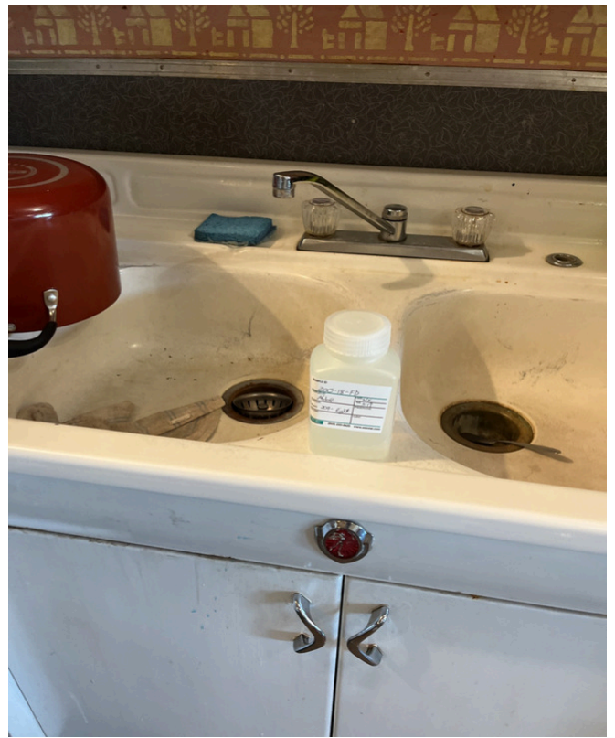
6/5/2024 - 200-18 - Malta Bend - Room 209 - Right
