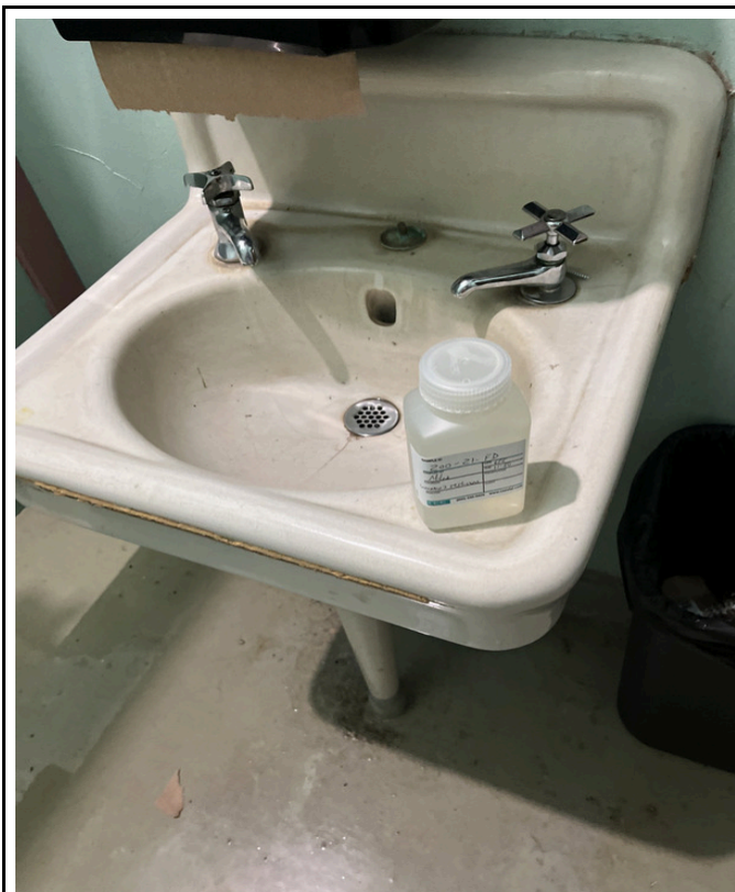
6/5/2024 - 200-21 - Malta Bend - Women's Restroom
