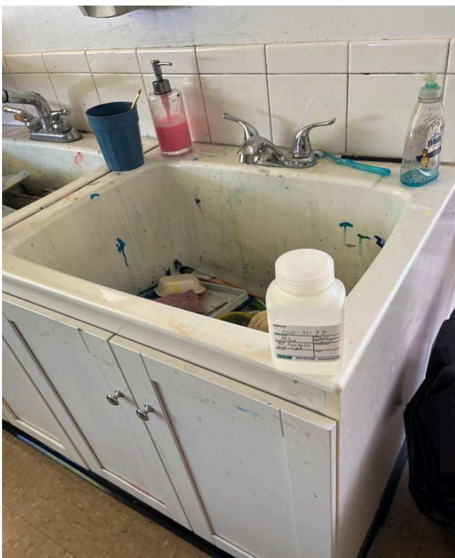
6/5/2024 - 200-31 - Malta Bend - Art Room Double Sink - Right
