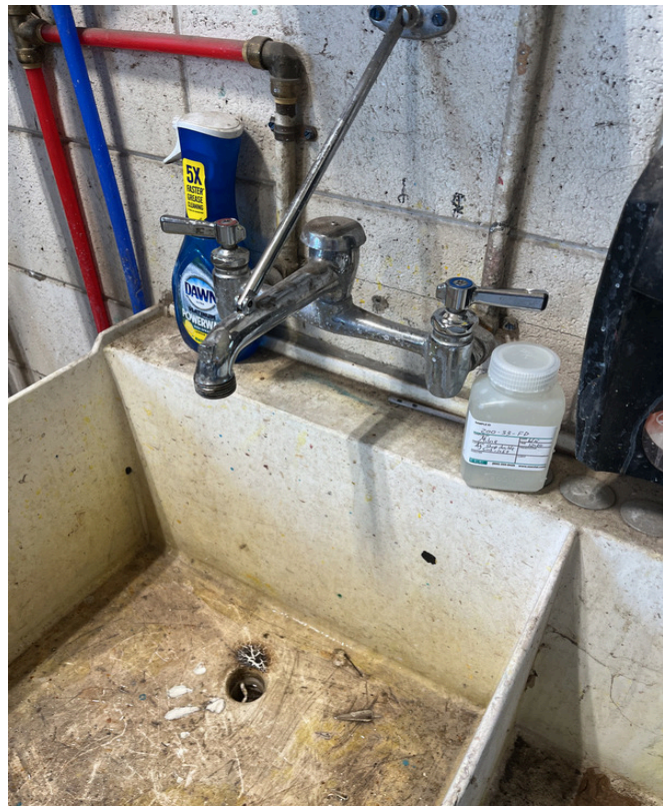
6/5/2024 - 200-33 - Malta Bend - Ag Shop Double Sink - Left
