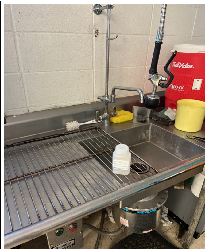
6/5/2024 - 200-1 - Malta Bend - Kitchen - West Wall - Right
