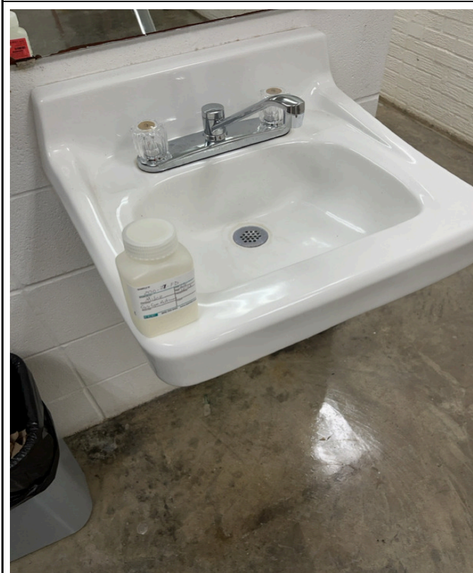
6/5/2024 - 200-27 - Malta Bend - Girls Gym Restroom
