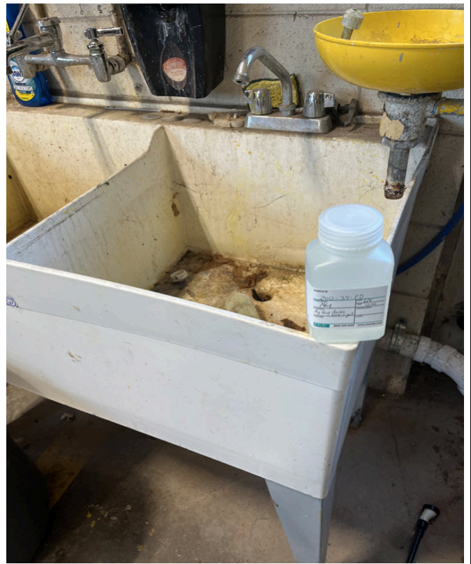
6/5/2024 - 200-34 - Malta Bend - Ag Shop Double Sink - Right
